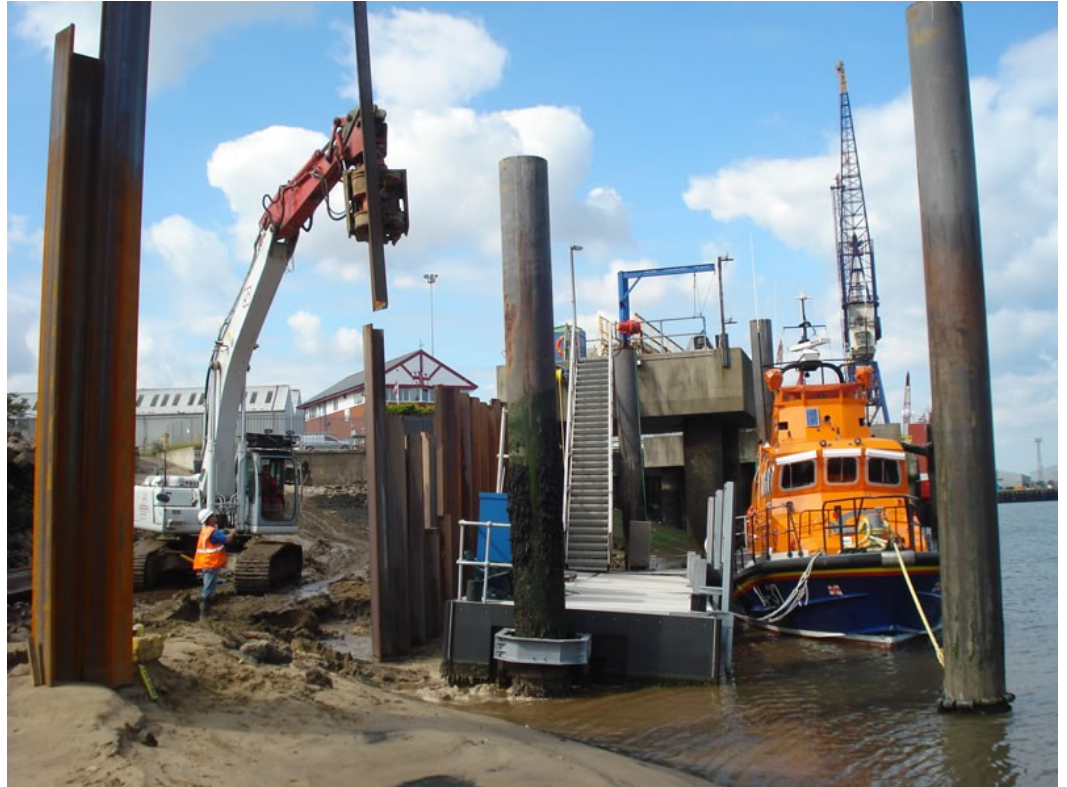
Working using the Movax
