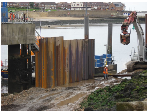
AU16 Sheet Pile Permanent Retaining Wall
