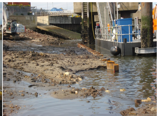
The Pile line at Finished Level
