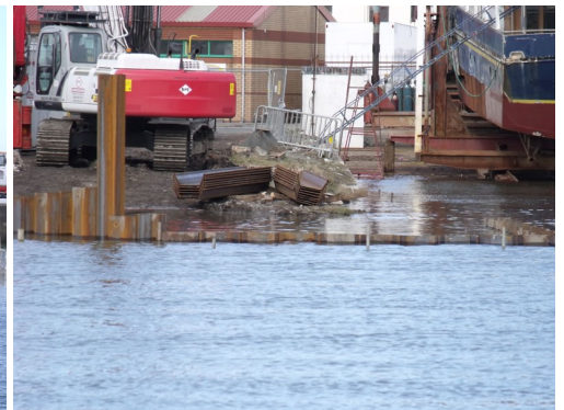
Piles are mostly below the tide line
