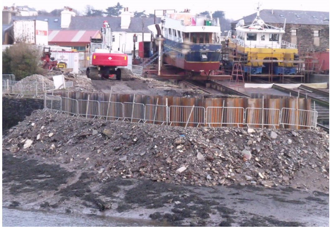
Piling Works Nearing Completion at Ramsay Shipyards
