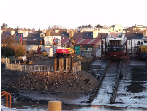
Starting Piling Works at Ramsay Shipyards
