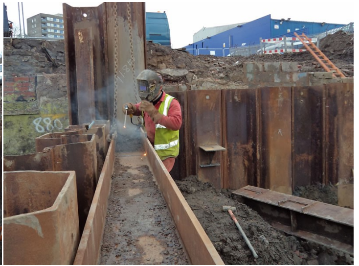
Welding the Steel frame
