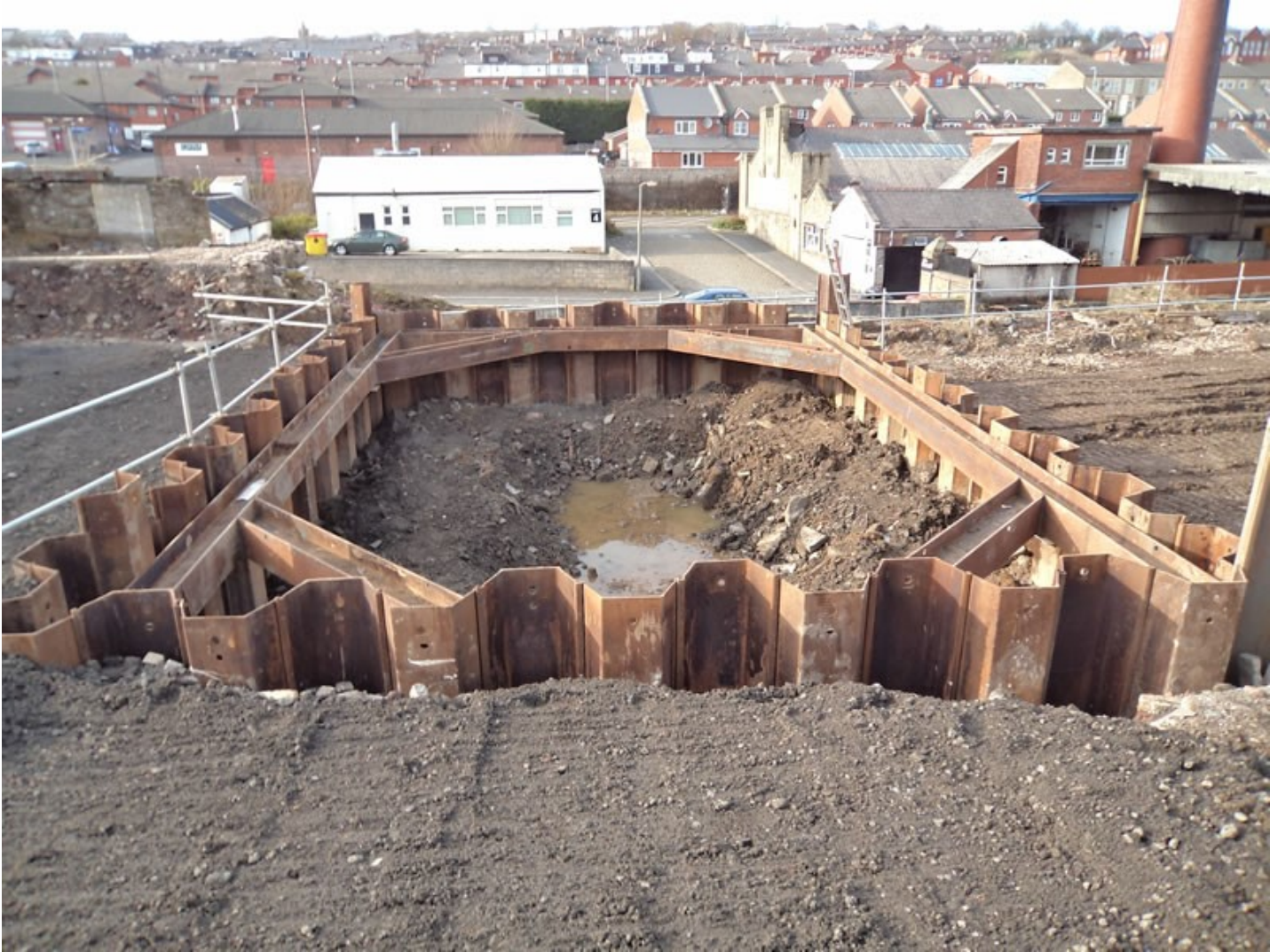
The Steel Sheet Cofferdam completed with its framework
