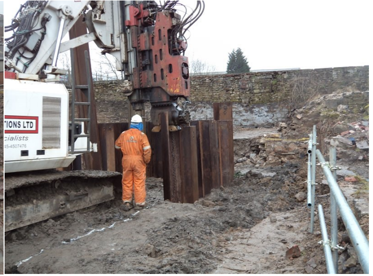
The Piles going down using a Vibratory Hammer
