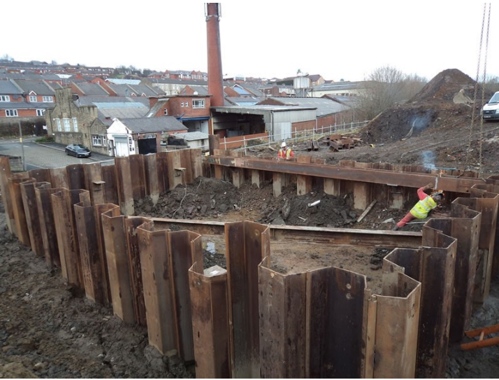
The temporary cofferdam all but completed
