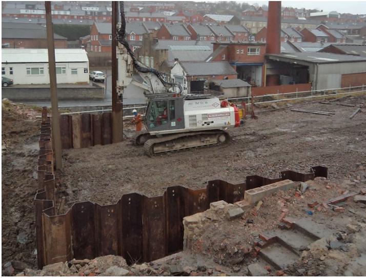
Piling the Cofferdam with the 13/16 Leader Rig
