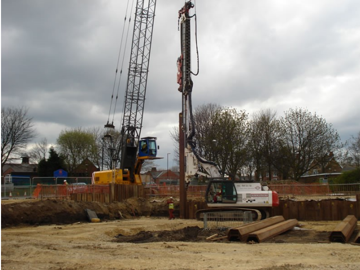
Piles are installed with our 13/16 Telescopic Leader Rig
