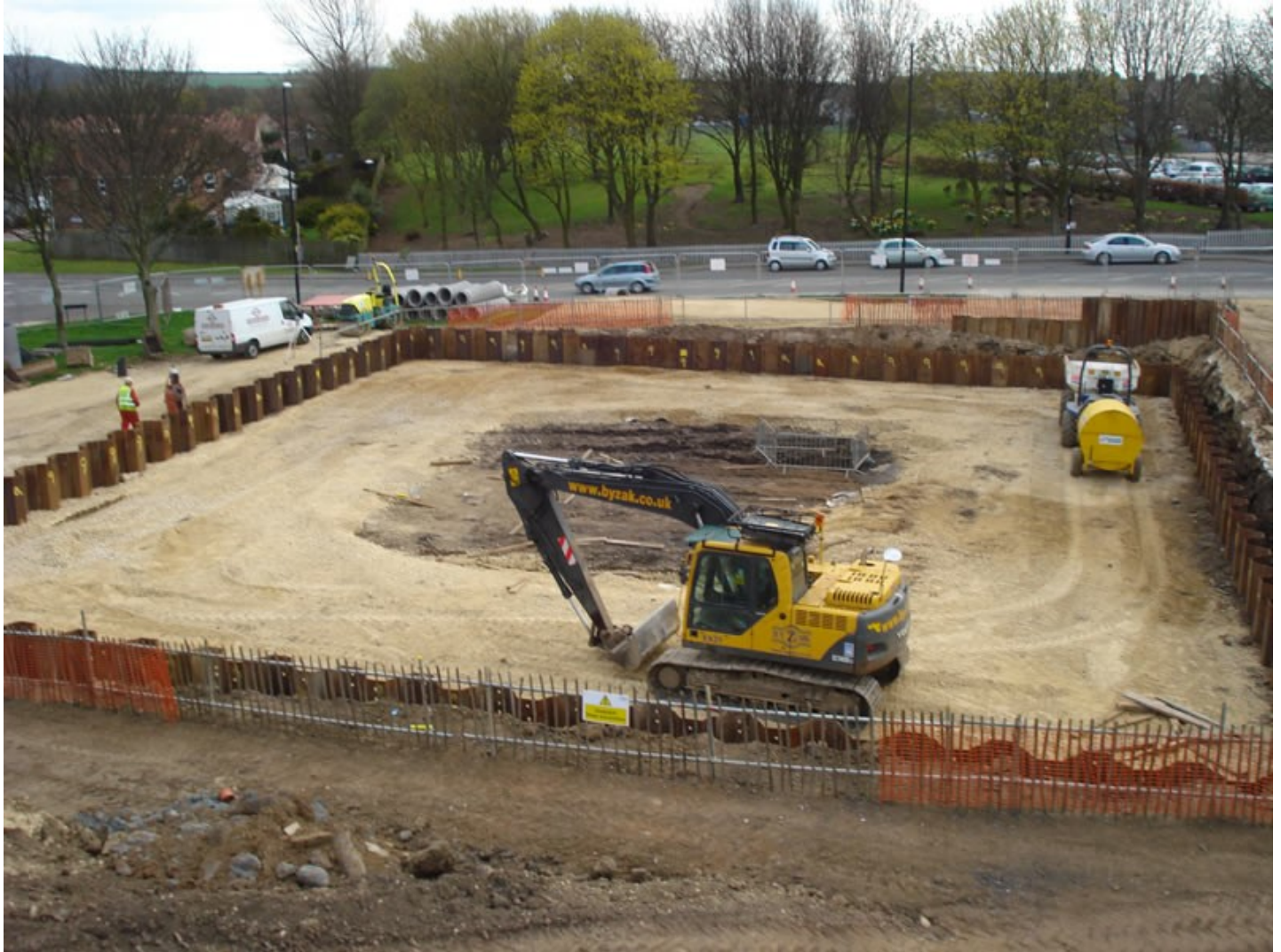
The completed cofferdam
