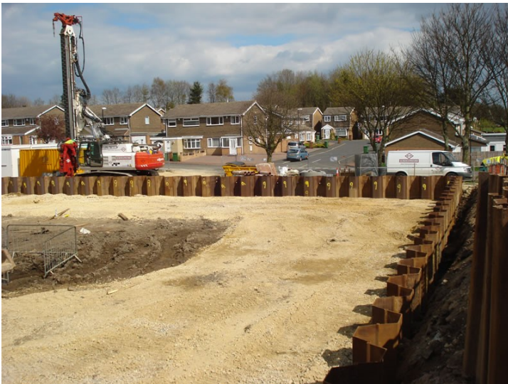
The last of the piles are installed
