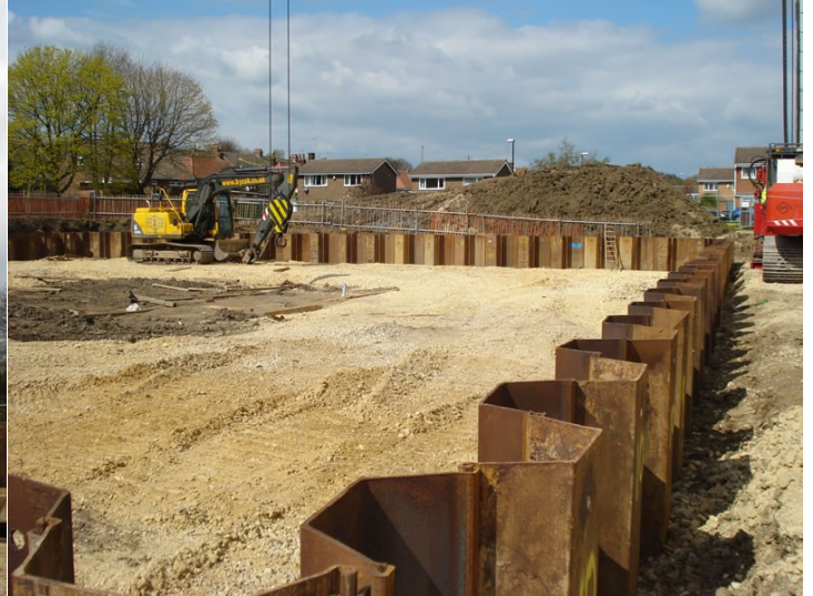
The pile line at Washington Tyne & Wear
