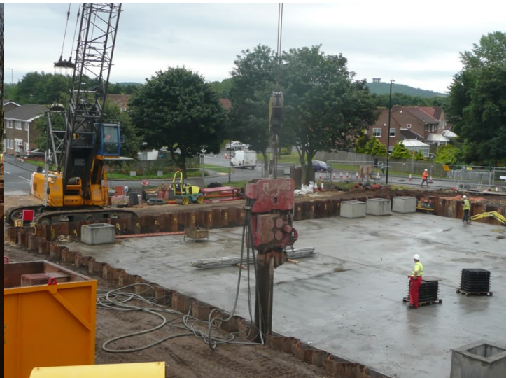
Extracting the piles now the storm tank has been installed underground
