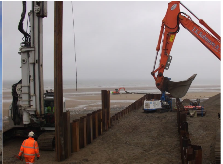
Temporary Pipe Trench
