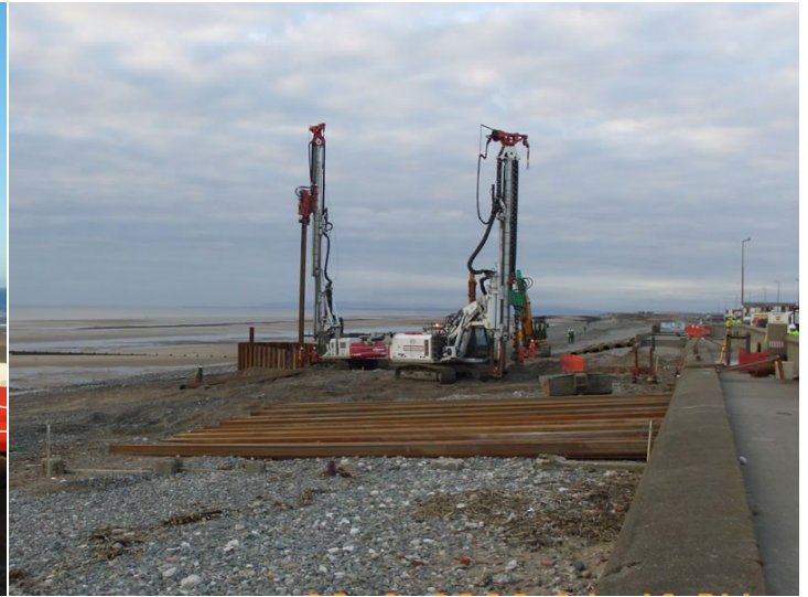
Piling the cable trench at Thornton Cleveleys
