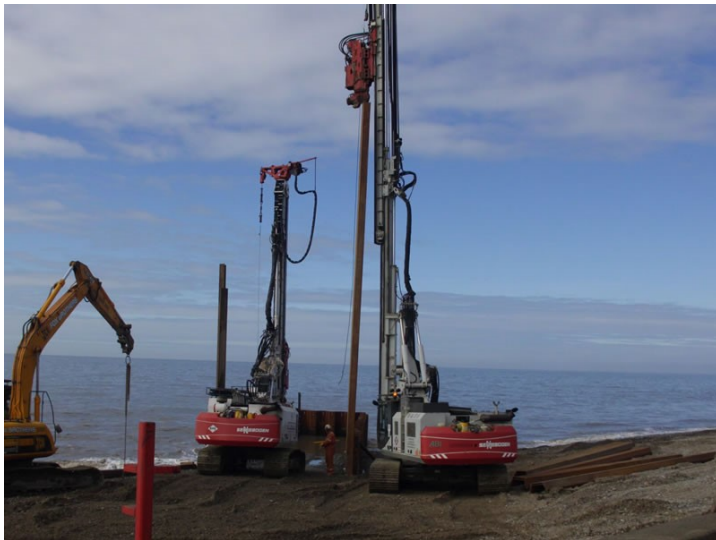
Piling until the tide turns
