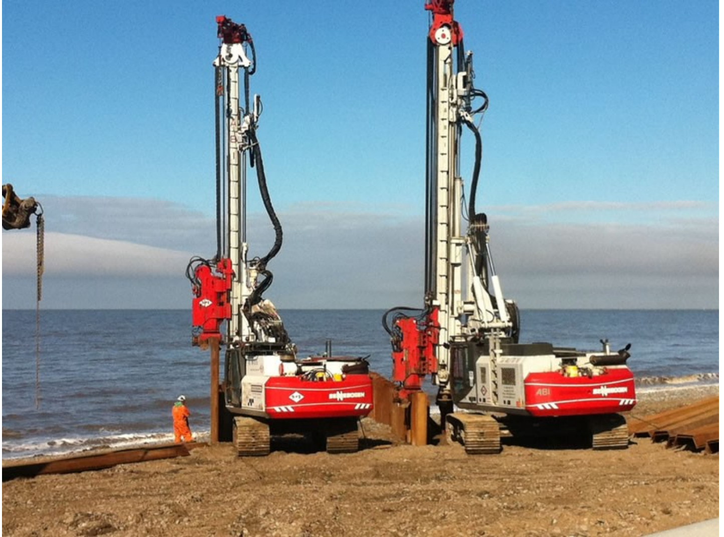
The twins (Leader Rigs) Piling in tandem
