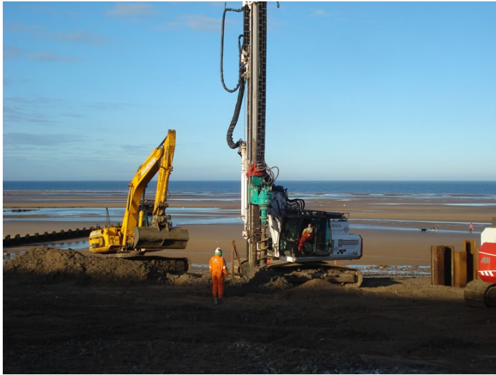
Auger Boring on the Beach
