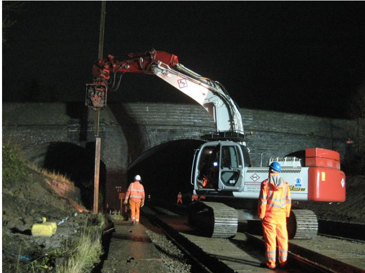
E385 Excavator with the Movax SPH75 Side Grip Vibratory Hammer
