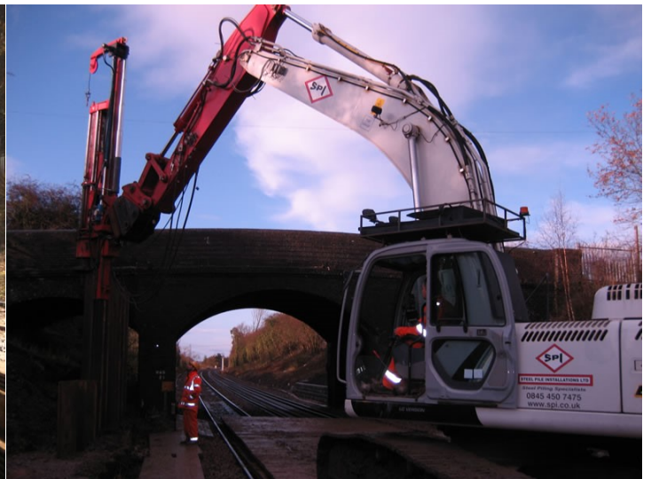
As daytime dawns the work continues under possession
