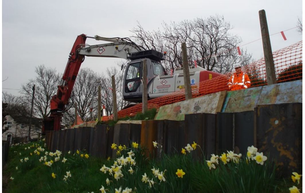
Installing the retaining wall with the Movax
