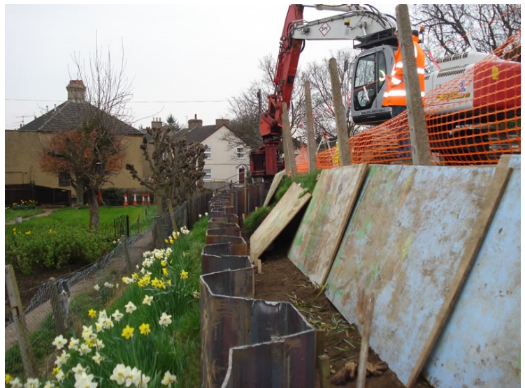
The Pile Line
