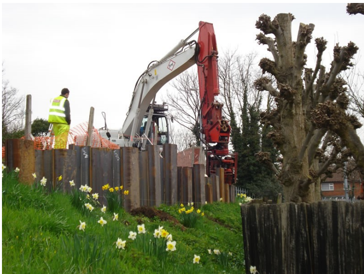
Piling for Bedfordshire Highways
