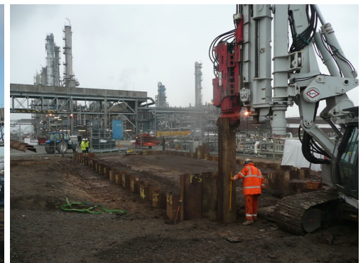
Cofferdam Nearing Completion
