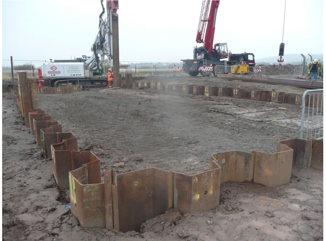
6 Sided Temporary Cofferdam
