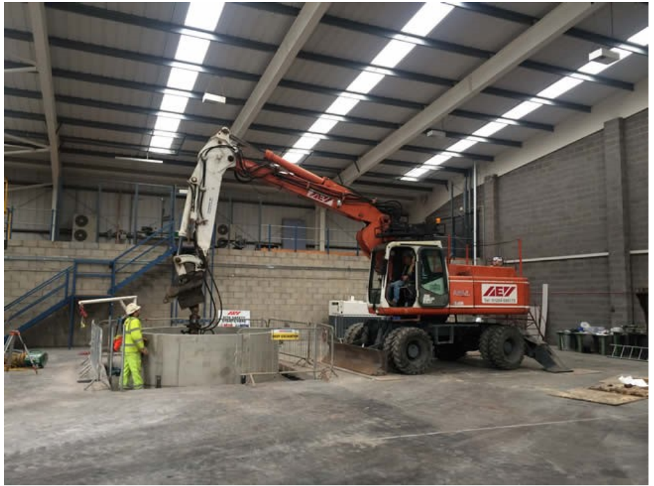
View at Floor Level
