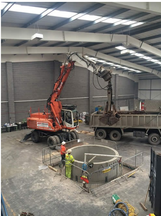
Excavation of Shaft
