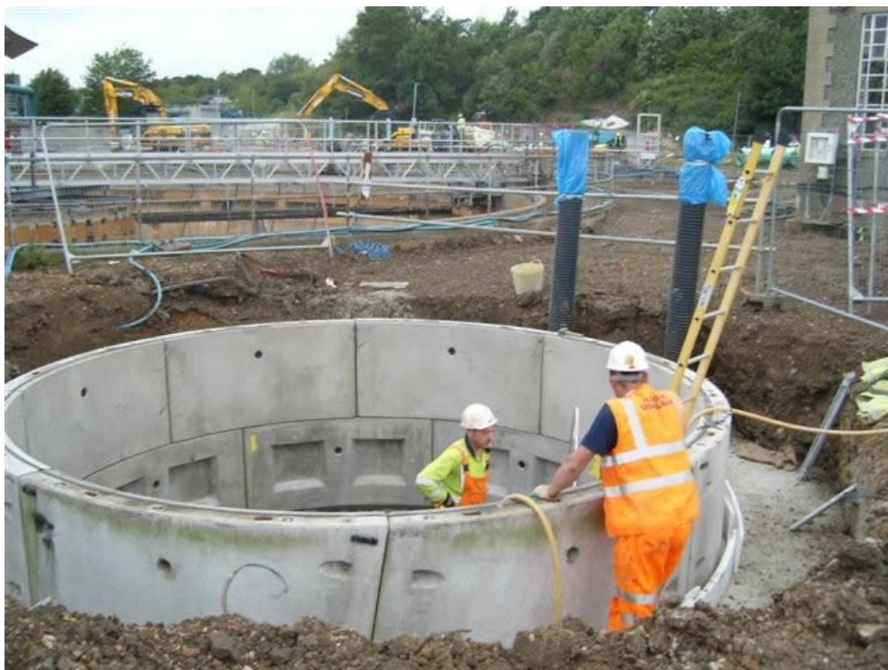
First two rings and collar built - ready to go
