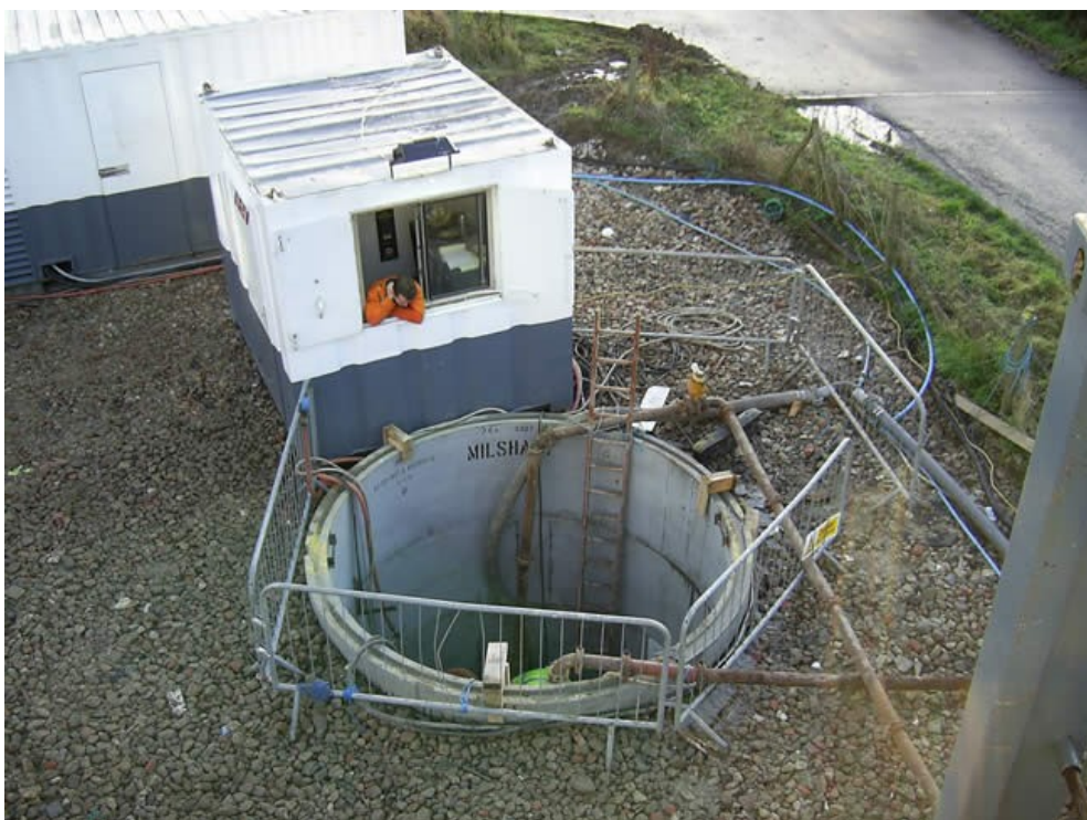
Full ring caisson complete
