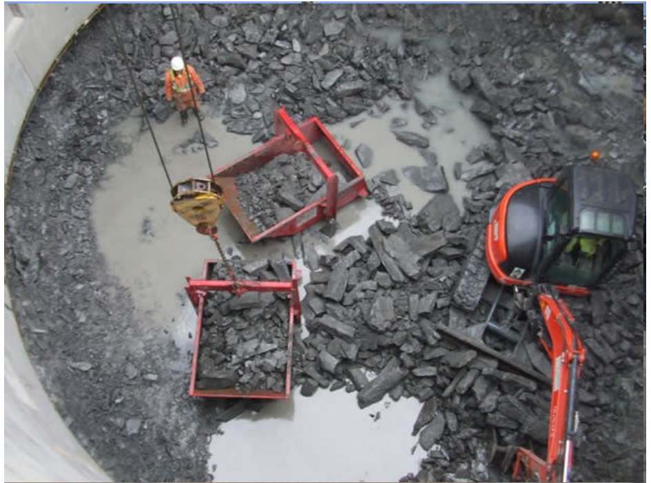
Excavation of Strong Mudstone
