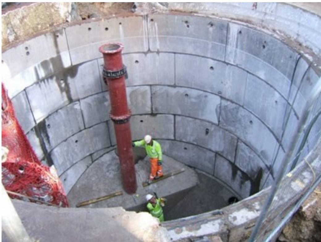
Partially completed shaft at Mill Brow Flood Alleviation Scheme, St Helens
