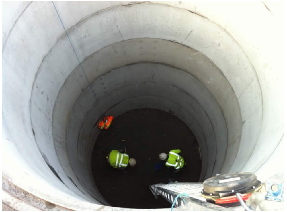
Excavation of the Shaft
