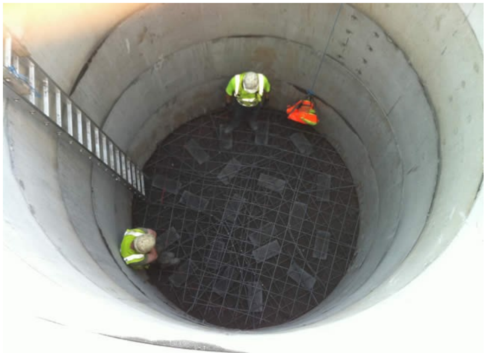
Base Reinforcement Fixed and Ready For Concrete
