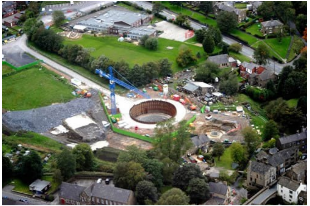
Aerial view of Denshaw Road works in Delph Lancashire
