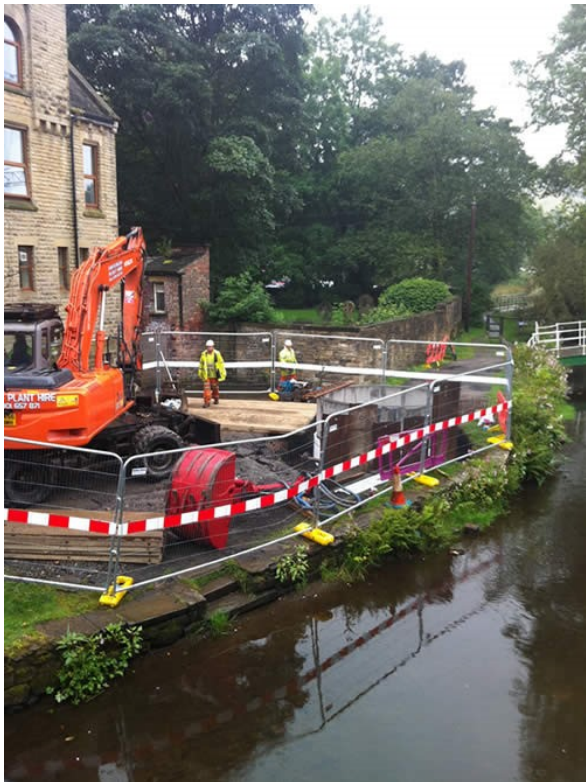
Shaft sinking between house and river at Delph
