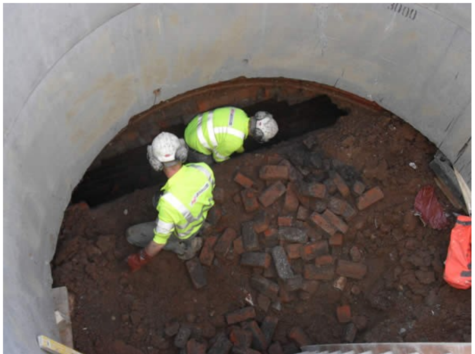
Dealing With the Existing Sewer
