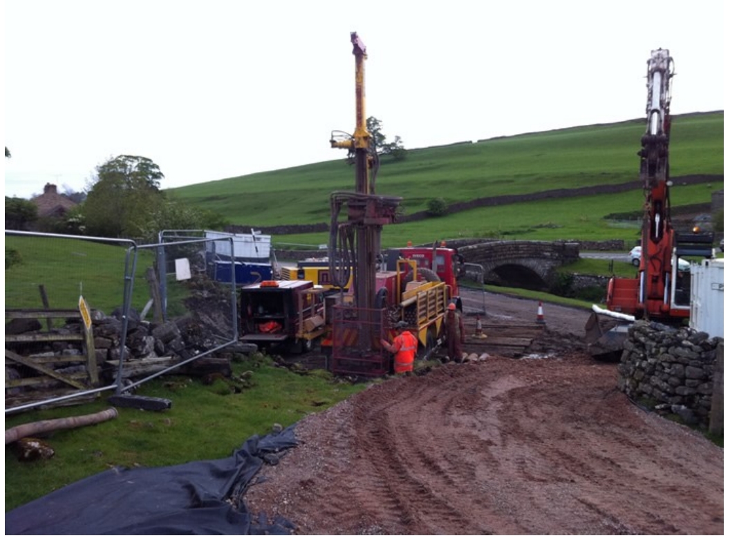
Shaft Sinking & Microtunnelling Project at Colby FTS, Cumbria for United Utilities
