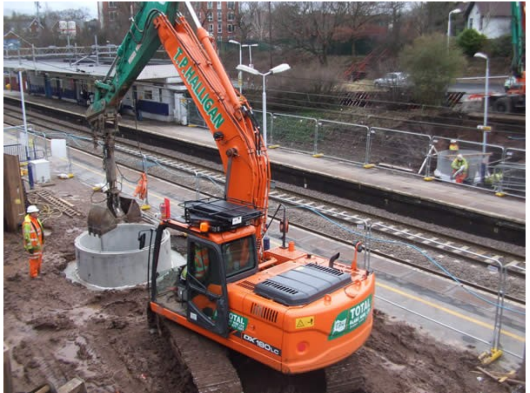
Shaft Sinking at Heald Green Station
