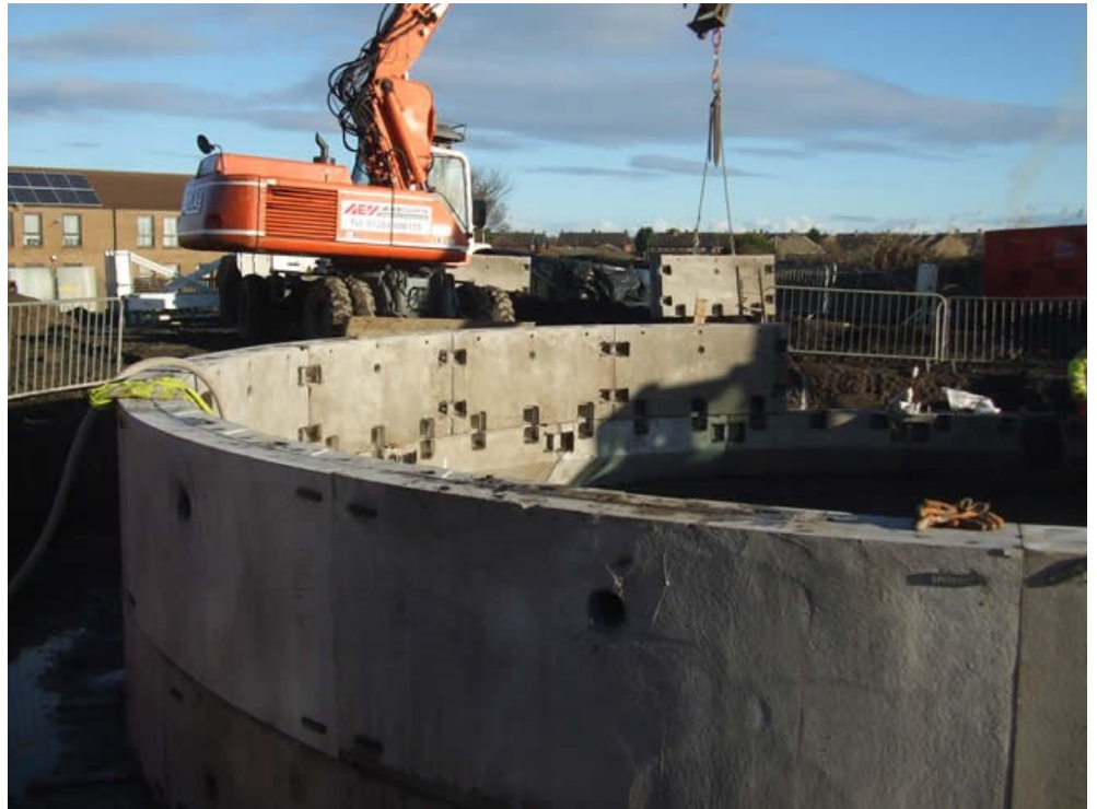
Shaft Sinking works underway at Wellwood Street, Amble
