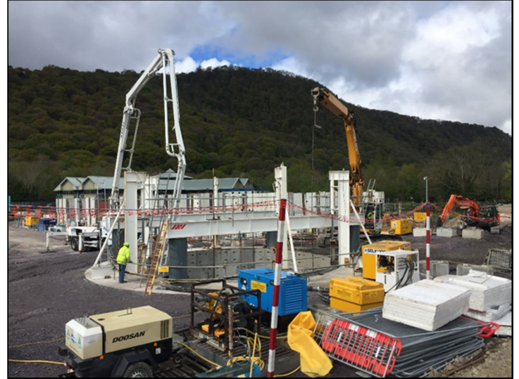
Surface Set Up Including Jacking Gallows and Suspension
