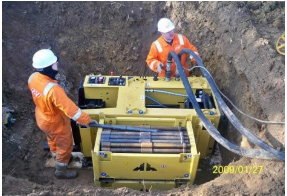
Pipe Bursting on site at YMCA Postley Road, Maidstone
