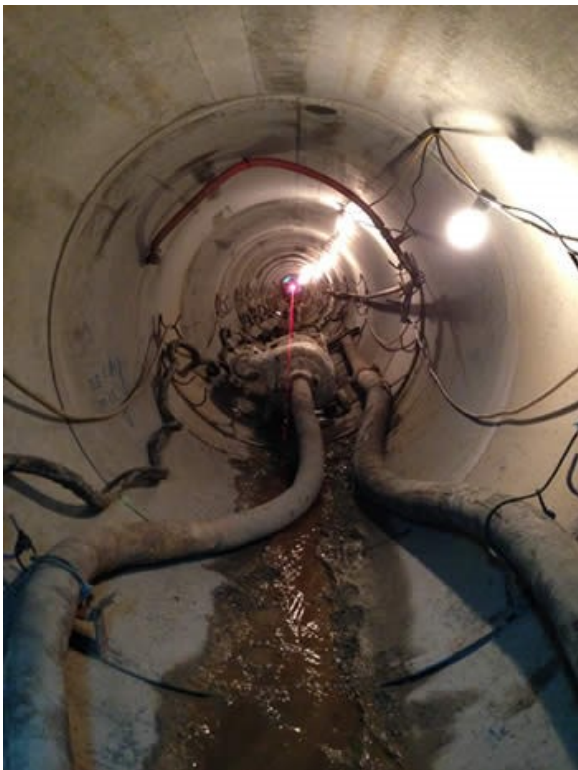
View along the tunnel
