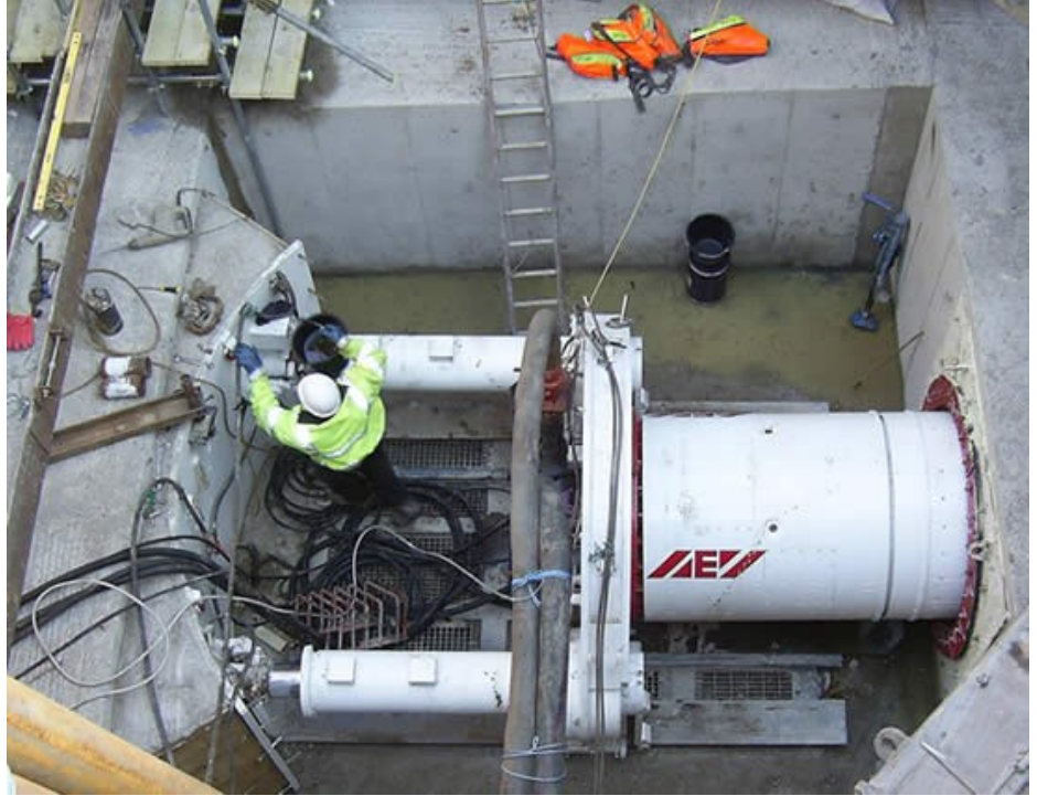
Microtunnelling Machine Being Launched
