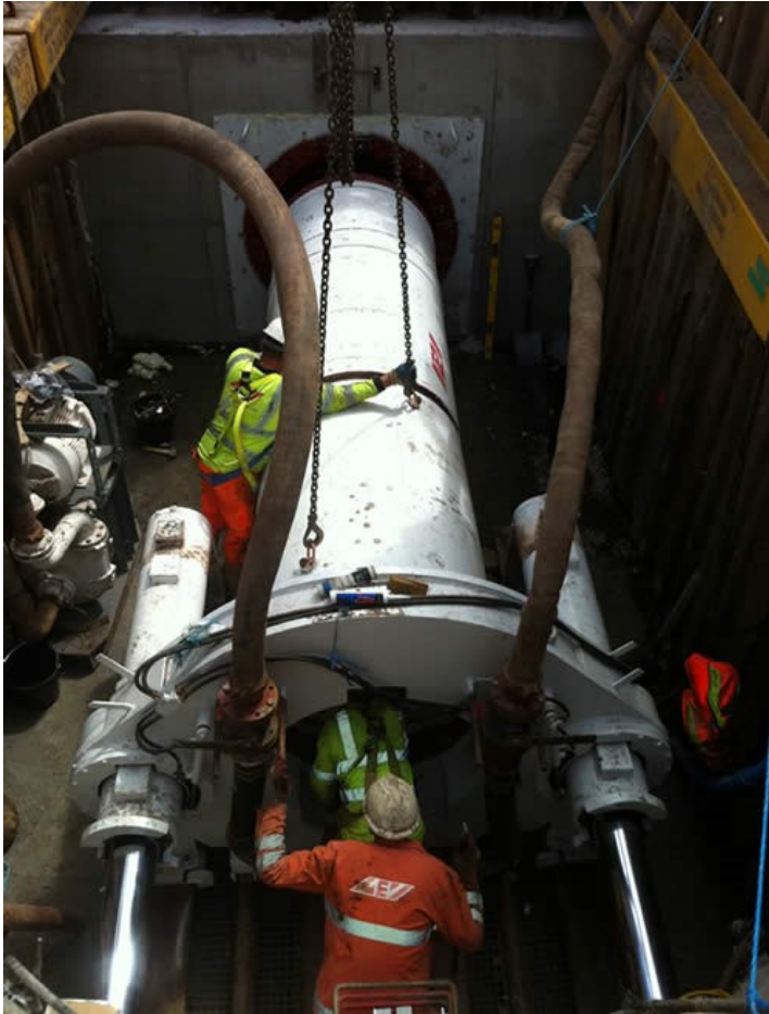
TBM ready to launch on site
