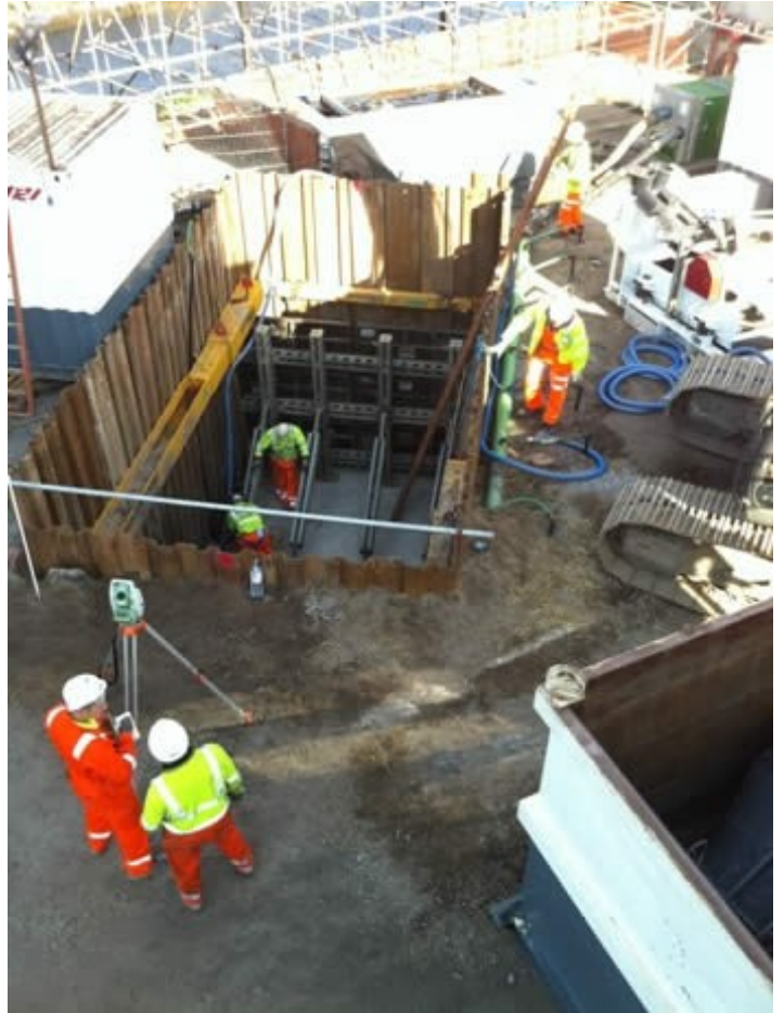
Drive pit set up at Ineous Chlor
