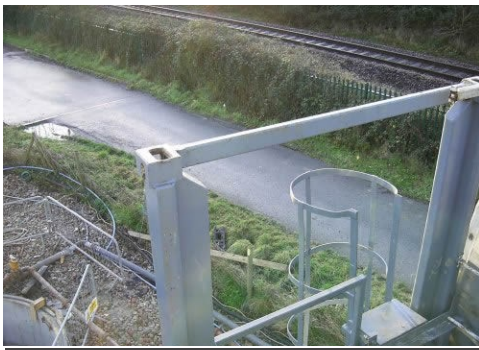
Drive Pit close to Railway Lines
