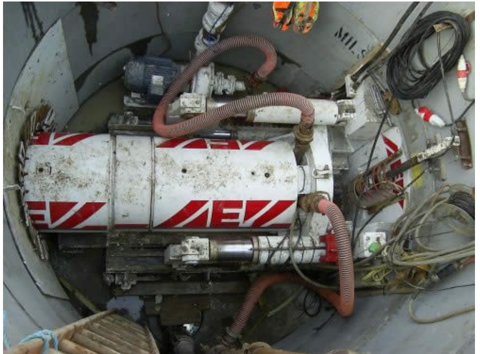
DN600 Iseki Unclemole Being Launched
