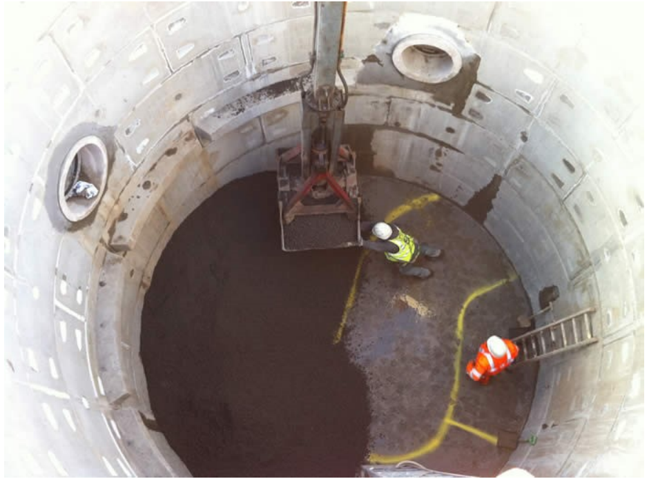
Shaft Finishing Works
