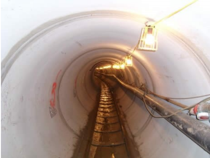
Completed Curved 1800mm ID Tunnel (viewed upstream)
